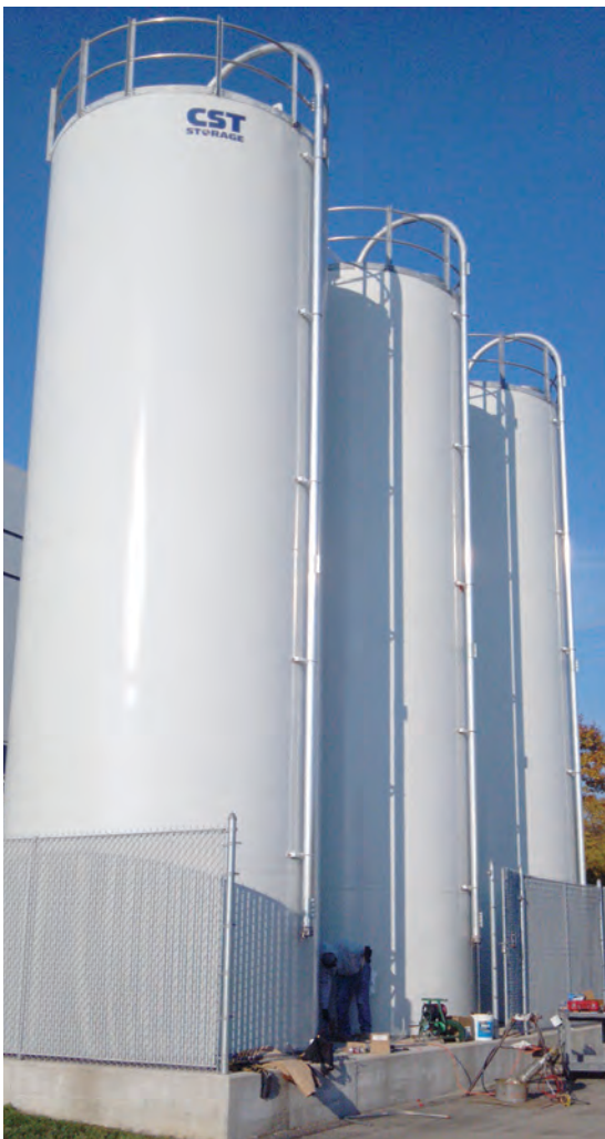
(3) 12' x 48' Factory-welded and epoxy-coated tanks for plastic pellet storage.
