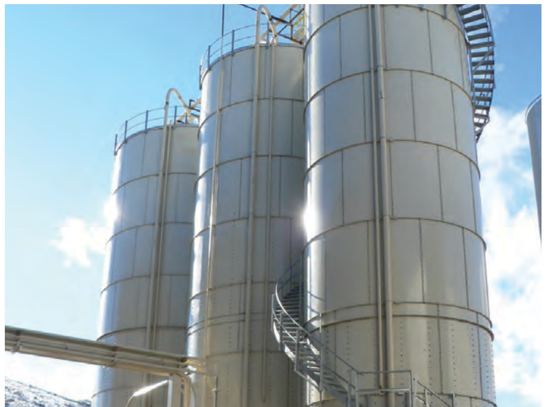
(3) 38' x 128' bolted tanks being built for a transload facility each storing 5,000 tons of sand.
