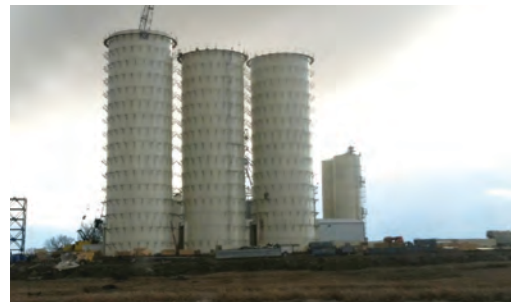
(3) 38' x 128' bolted tanks being built for a transload facility each storing 5,000 tons of sand.
