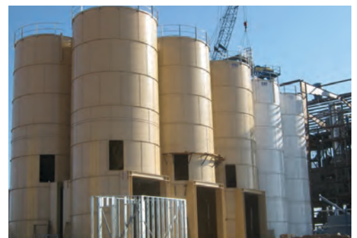
21' x 56' - 500 ton truck loadout silos shown here in 6 & 8 pack configurations.
