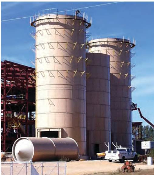
Standard 24' x 80' each storing 1,000 tons of frac sand.
