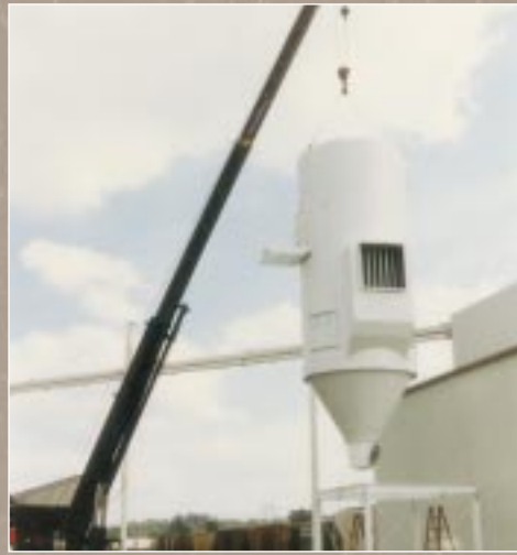
MCF Filters can be shipped fully welded to simplify and speed installation.
