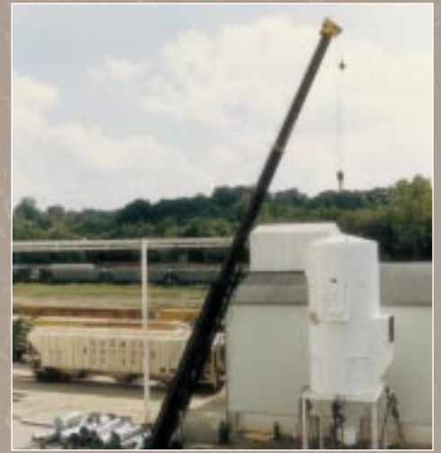
MCF Filters can be shipped fully welded to simplify and speed installation.
